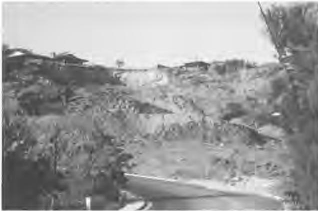
Figure 17. Truman Drive landslide on the south side of the Santa Clara Bench; failure occurred in the Petrified Forest Member of the Chinle Formation.
