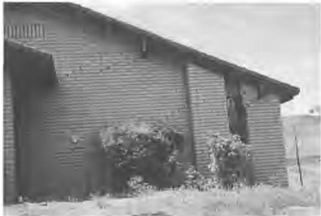
Figure 14. Cracks in the wall of a home on the Santa Clara Bench caused by expansion of the underlying Petrified Forest Member of the Chinle Formation.
